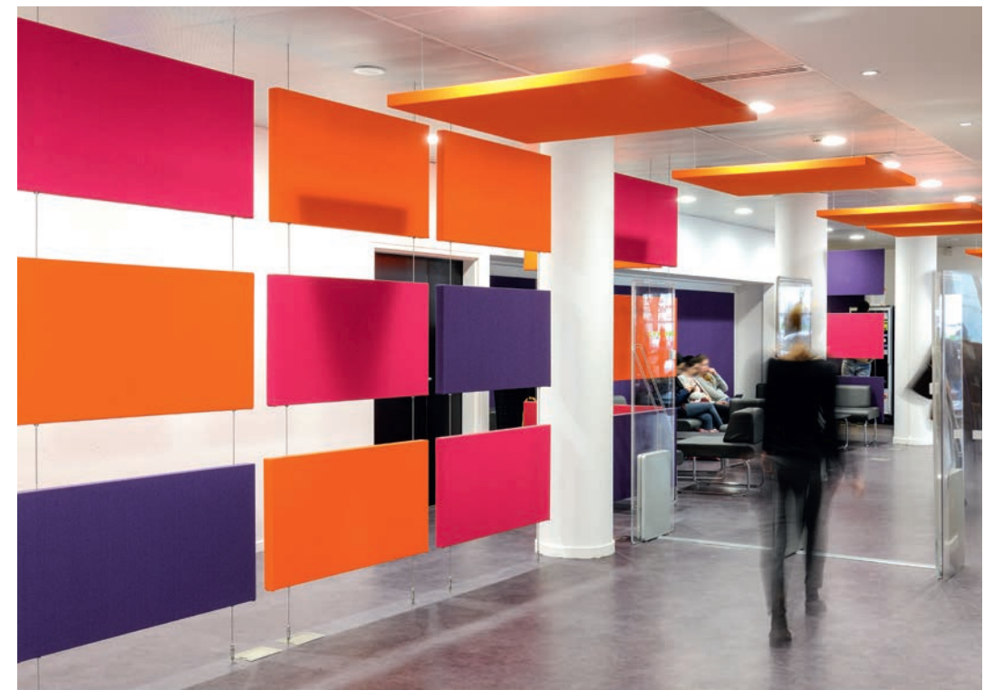
Stereo panels mounted on cables that pass through them and are anchored to the floor to achieve a partition. Chevreul library of Lumière Lyon 2 University. Architects: Alain Lelievre and Nesso Architects, 2017.
