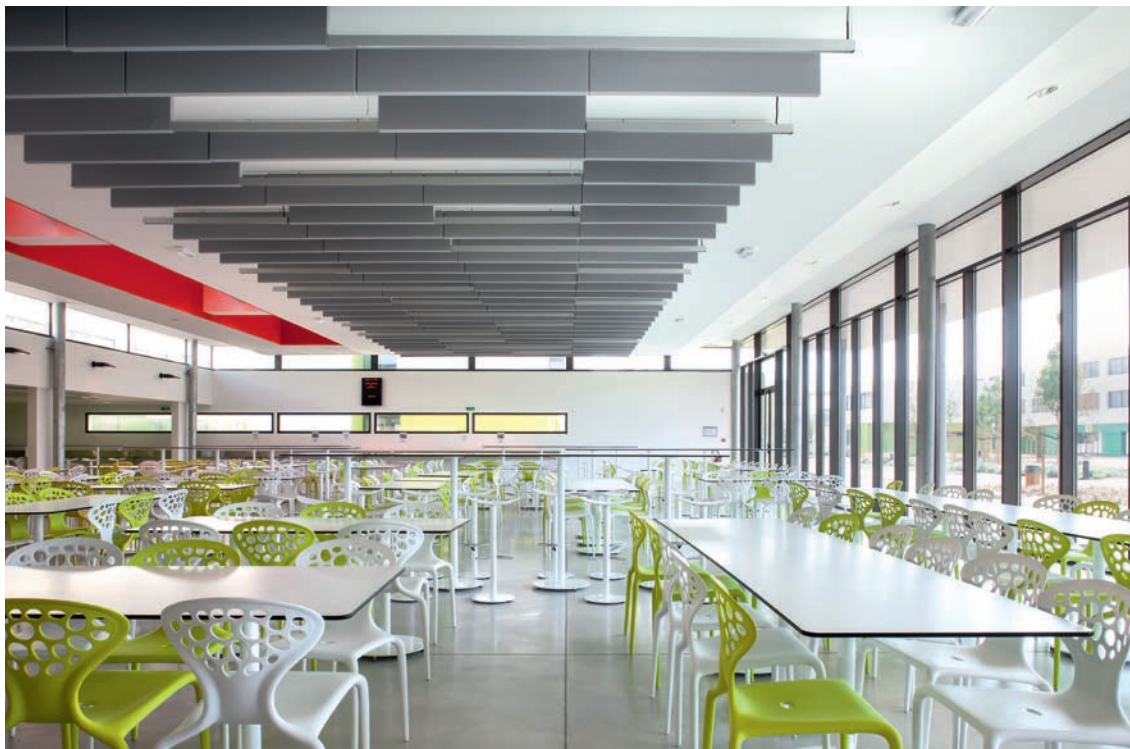
Stereo panels as screw-mounted baffles, a special project request. Canteen of the Victor Hugo secondary school in Lunel, southern France. Architect: Pierre Tourre, Montpellier, 2009.
