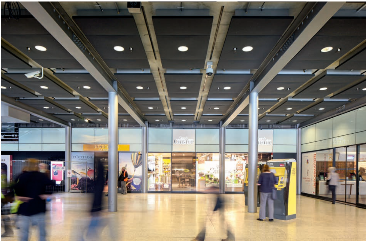
Special project: Stereo panels fitted on sliding runners to enable access to lighting and sprinkler systems. Saint Lazare station in Paris. Architects: SNCF Gares et connexions, Arep, DGLA, 2012.
