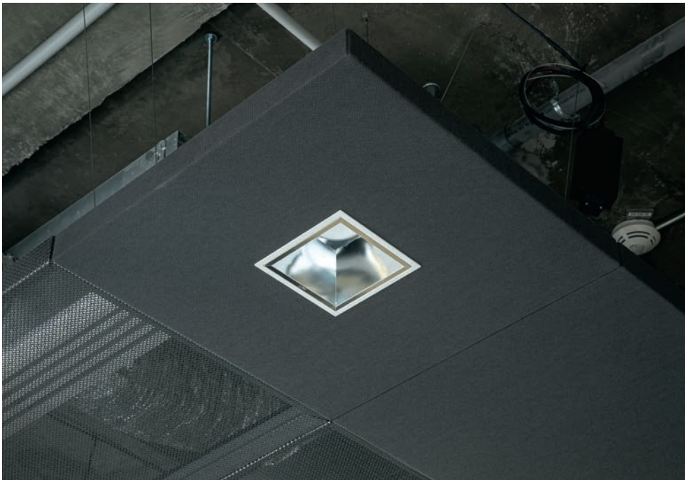
Optional recess in an absorber panel, in this case for a light.
